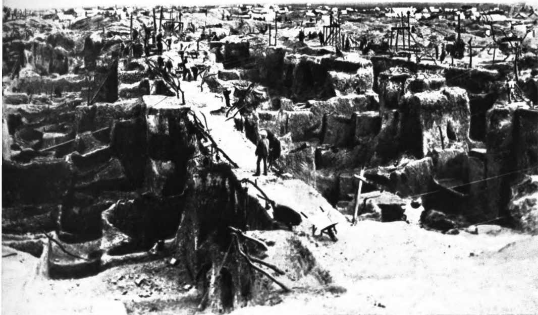
53 The Kimberley mine in early 1872, showing the varying depths of the claims and the roadways between them
